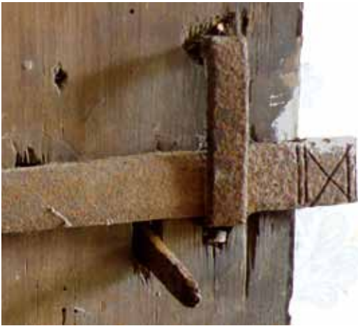
Fig. 13. An X-mark on the latch of a cellar door, about 1720.
